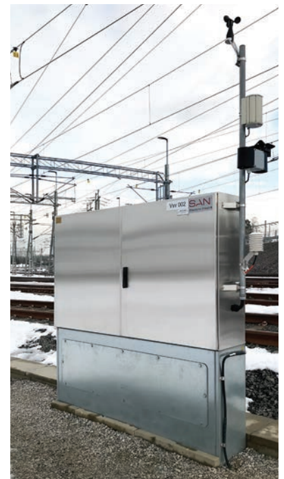
Control cubicle enclosures are available in stainless steel, painted steel, or reinforced fiberglass.
