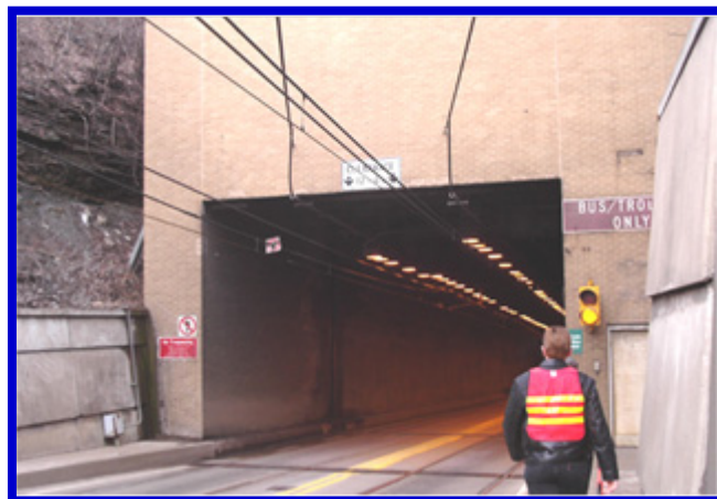
Pittsburg – Mt. Washington Tunnel Portal
